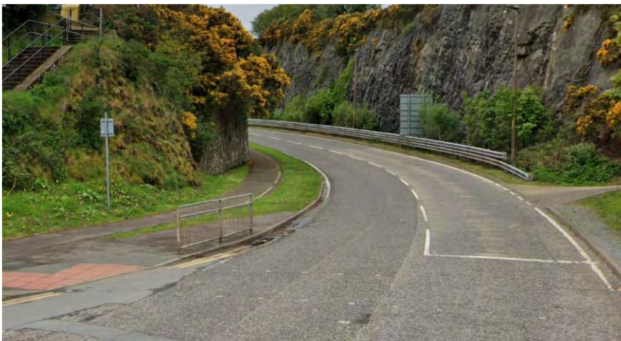
Photo 9D: Immediately west of the crossroads a shared pedestrian and cycle route starts. The sign on the left indicates that the cycle route ends, but there is no corresponding sign to indicate that it starts here. It is recommended that a shared use sign indicating the mandatory cycle route facing the crossroads is installed here, and painted on the surface of the route.
