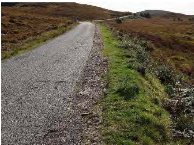
Photo P: (5km) Single track section of C1221 is provided with passing places, but clearly traffic often uses the verge. While this does cause damage, it also keeps vegetation short and suitable for pedestrians, although rather rough.
