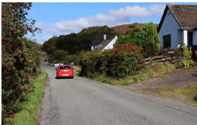
Photo F: (2.5km) Single track in Badicaul. As can be seen from the photo, the single-track road is wide enough for a vehicle and a marginal strip reserved for pedestrians and cyclists. Passing places are not defined but could be made more obvious for drivers with the use of white edge marking and statutory signage.
