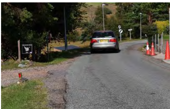
Photo Q: (5.3km) Single track pinch-point in C1221 at Drumbuie, with inadequate passing place and nowhere for pedestrians to walk apart from a narrow strip of verge regularly used by vehicles as a passing place. Beyond this (left of car in photo) an informal path leads down the bank to the bus shelter, the roof of which is just visible.
