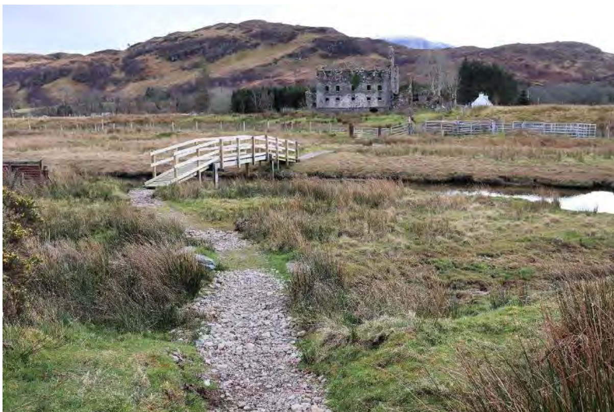
Photo: After passing the Barracks the path descends gently to a bridge over the old course of the river (point D on map). Ramps onto the bridge were installed in 2021. Gravel surfacing is dug locally.
