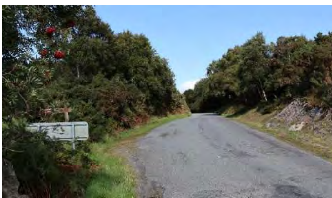
Photo G: (2.6km) At the north end of Badicaul the C1232 is briefly double then narrows to a pinch point with poor visibility and virtually no verge on which pedestrians and cyclists can find refuge. At this point a recreational path leads to the shore, and immediately beyond this an informal path has been created through the woodland to avoid this section. This is recommended for improvement and signage in the first section of this report.
