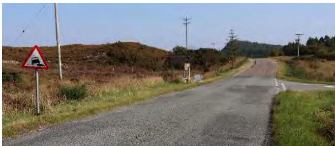
Photo U: (6.7km) Double track section of C1221 north of Drumbuie shows a wide verge as far as the junction with the road to Achmore, C1222, beyond which it is single track, the verge containing a hidden gully leading to a culvert which poses a hazard to road users, especially pedestrians.
