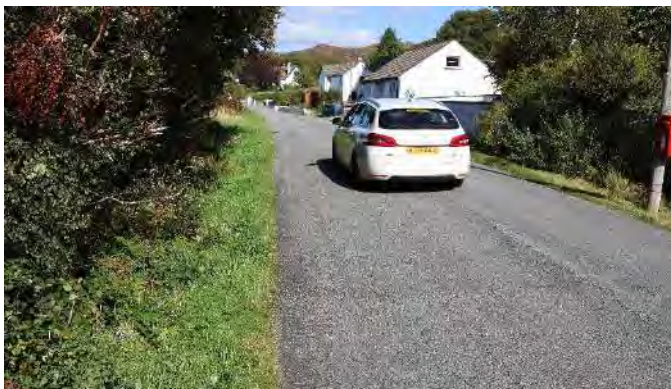
Photo D: (2.2km) A pinch point opposite the posting box occurs where the verge is too narrow to walk on, and even if the vegetation was cleared, a deep gully prevents causeway widening. Construction on the verge or a pedestrian priority zone demarcated by white lining would be necessary here.
