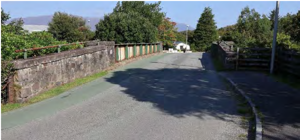
Photo BB: (8.7km) The railway bridge in Plockton has an unexplained strip of green tarmac. The footway finishes on the east (right) side, so any pedestrian, cyclist and wheeling travel should be accommodated on that side or provided with a pedestrian-controlled crossing. White line road marking would assist road safety here.
