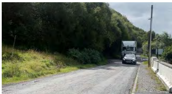
Photo I: (3km) Narrow double-track section of C1232 in Erbusaig is in places provided with a roadside footway of loose gravel construction.
