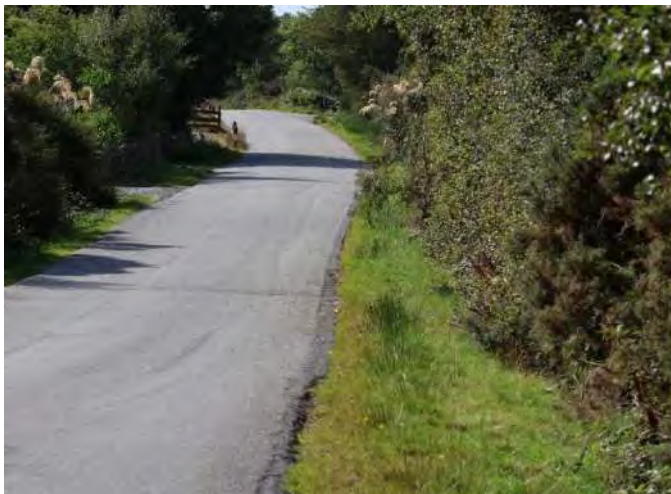
Photo L: (3.6km) Broad single-track section of C1232 in Erbusaig has the potential for a pedestrian footway on the west (right) side if the vegetation was cleared back and the surface maintained adequately.
