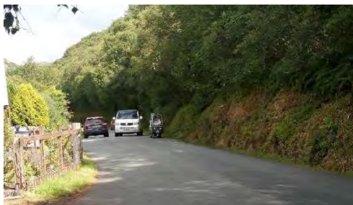
Photo H: (2.8km) Congestion at the pinch point by the Erbusaig Cascade. Single track road is similar to that in Badicaul with a large drop on the left protected by a low stone wall, and with no opportunity for carriageway widening. A similar solution might be appropriate: Partition the road with a white line, reserving a one-metre-wide section for pedestrians and cyclists and providing passing places.
