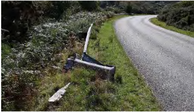
Photo N: (4.1km) Double track section of C1221 with ample room on verge for pedestrians. Requires further cutting back of vegetation and adequate maintenance of surfaces. Also requires repairs to crash barrier.
